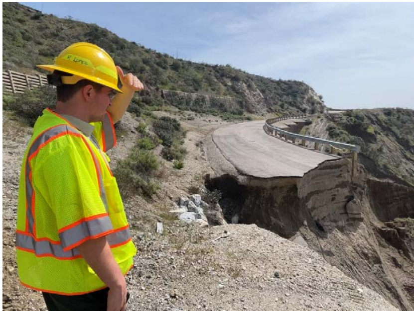
United States, 2023. Inspection of a storm-damaged roadway in California. Credit : Andrew Avitt / USDA Forest Service, Public Domain.
